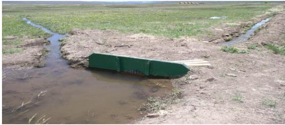
**Fig. 5. Example of a headgate used for diverting water in a mountain meadow. Differing numbers of board slats are placed in the slot on the face of the structure to control how much water flows into each of the ditches. (Photo by John Scott)**
